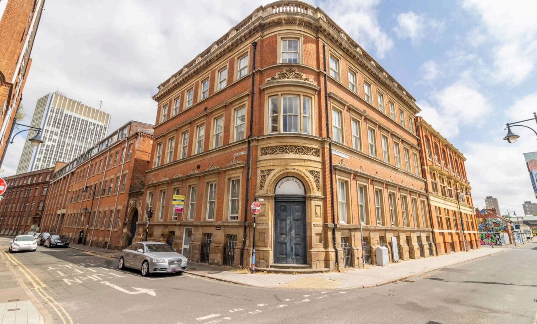
Flat 3, Wimbledon House, 21 Wimbledon Street Leicester
